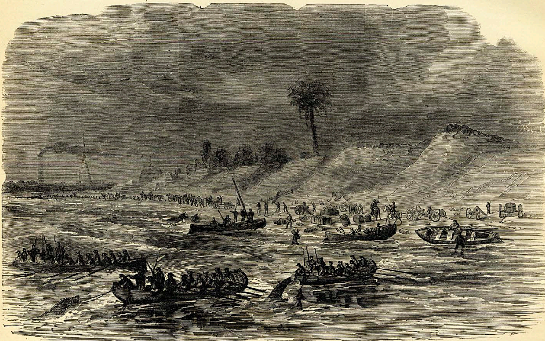
LANDING REINFORCEMENTS ON SANTA ROSA ISLAND.
