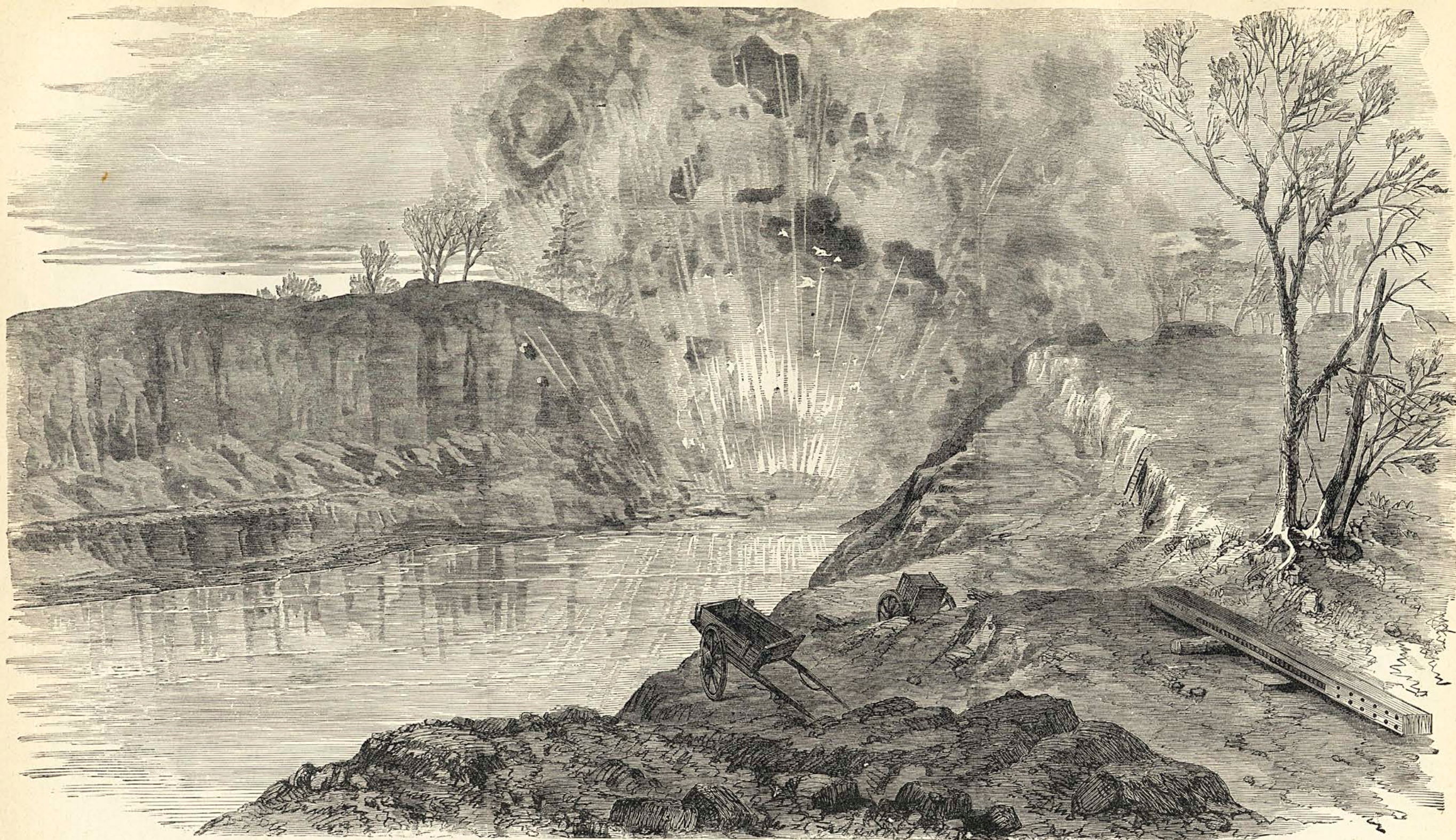
BLOWING OUT THE BULKHEAD OF THE DUTCH GAP CANAL.
