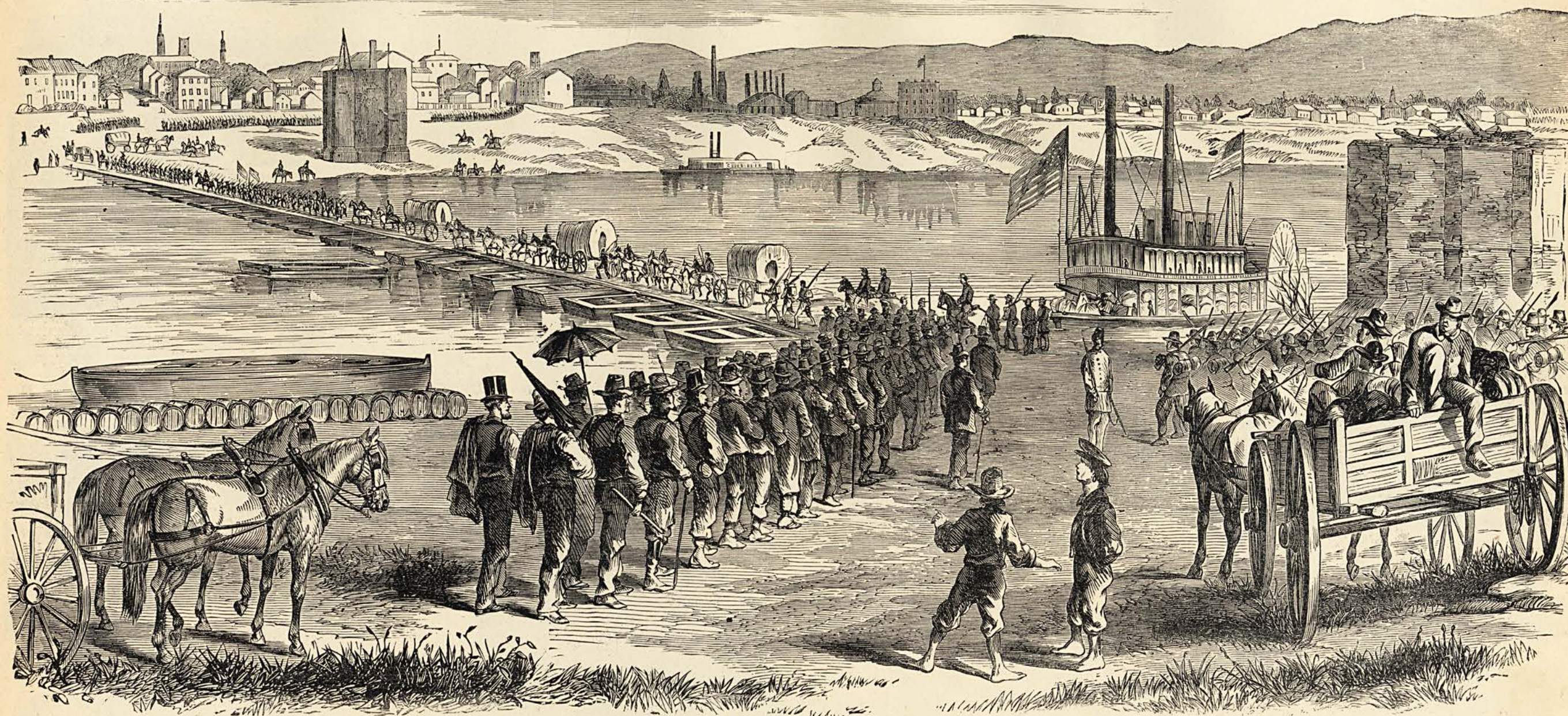
VOLUNTEERS FOR THE FEDERAL ARMY CROSSING FROM CINCINNATI, O., TO COVINGTON, KY., ON A BRIDGE OF COAL-BOATS HASTILY CONSTRUCTED THAT THEY MIGHT DEFEND THE BORDER FROM THE INVASION OF GENERAL KIRBY SMITH.—FROM A SKETCH BY H. LOVIE.
