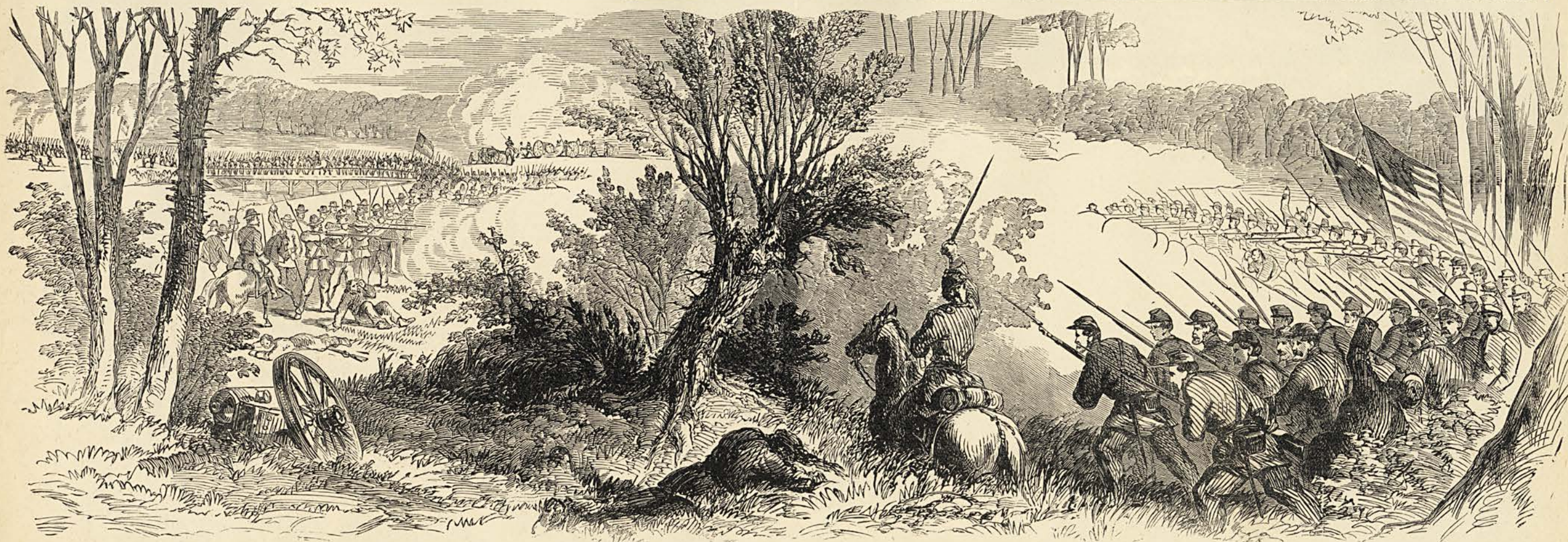
THE FEDERAL TROOPS, UNDER GENERALS BRENNAN AND TERRY, DRIVING THE CONFEDERATES, UNDER GENERAL WALKER, ACROSS THE POCOTALIGO BRIDGE, NEAR THE CHARLESTON AND SAVANNAH RAILROAD, OCTOBER 22, 1862.—FROM A SKETCH BY W. T. CRANE.
