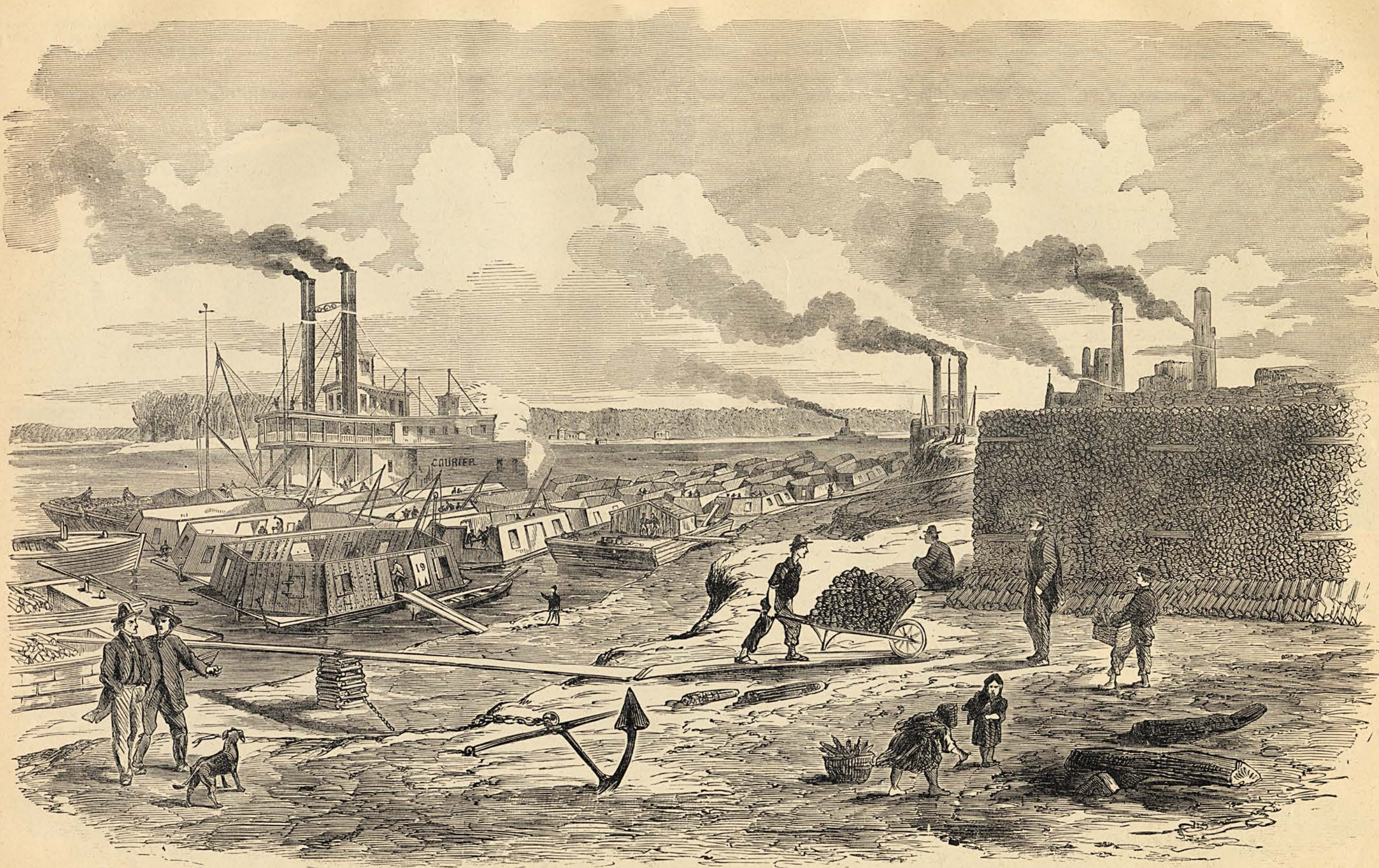
CONSTRUCTION OF FLOATING MORTAR BATTERIES BY THE FEDERAL GOVERNMENT, AT THE UPPER FERRY, ST. LOUIS, MO.
