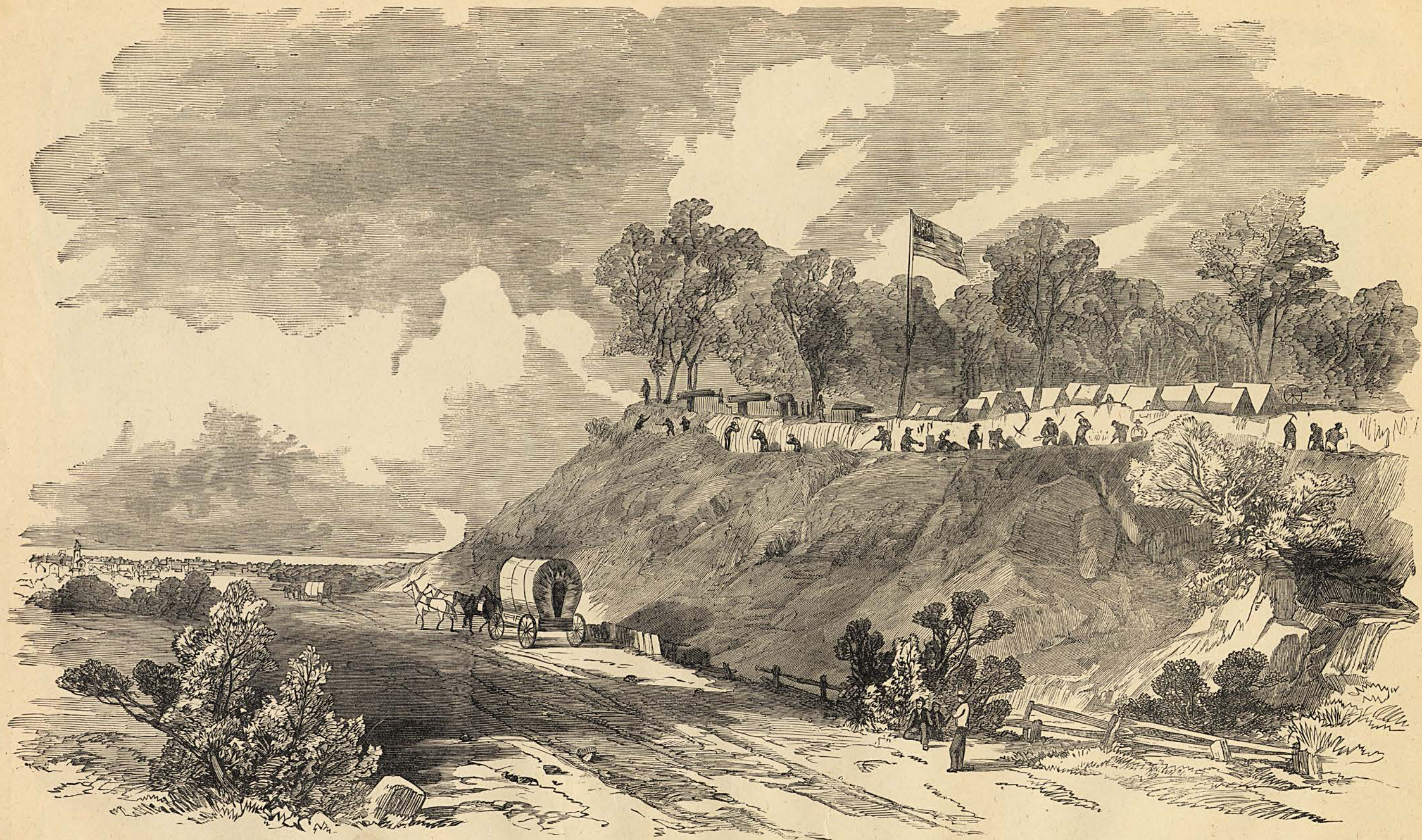
THE NAVAL BRIGADE, UNDER LIEUT. PERKINS, CONSTRUCTING THE MARINE BATTERY ON SHUTER'S HILL, TO GUARD ALEXANDRIA, VA., AND TO COMMAND THE FAIRFAX ROAD.
